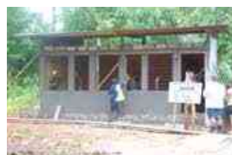
Figure 1. Constructing a new kindergarten
