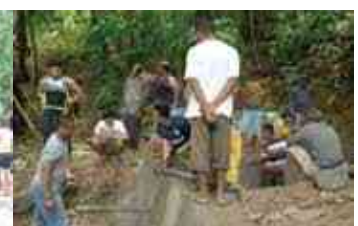
Figure 2. Constructing a water tub
